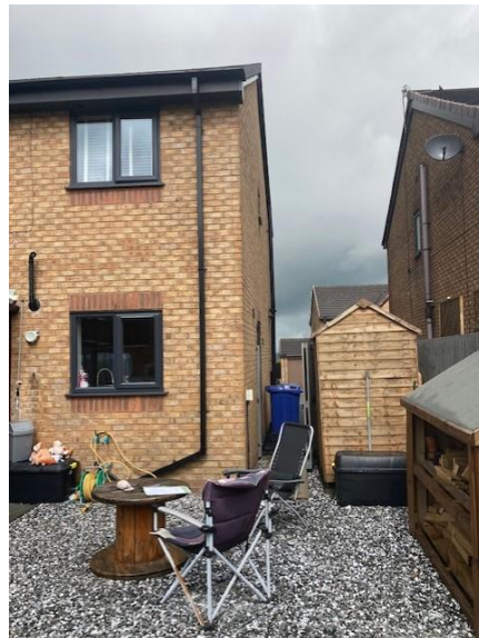
Photo 2: rear elevation gap with No. 50
